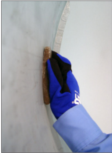
F-1 The dolly is being used as a backup tool for a hammer blow to the opposite side of the panel.
