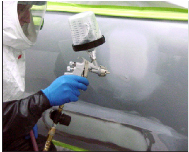
C-1 A primer may be recommended before body filler is applied.
