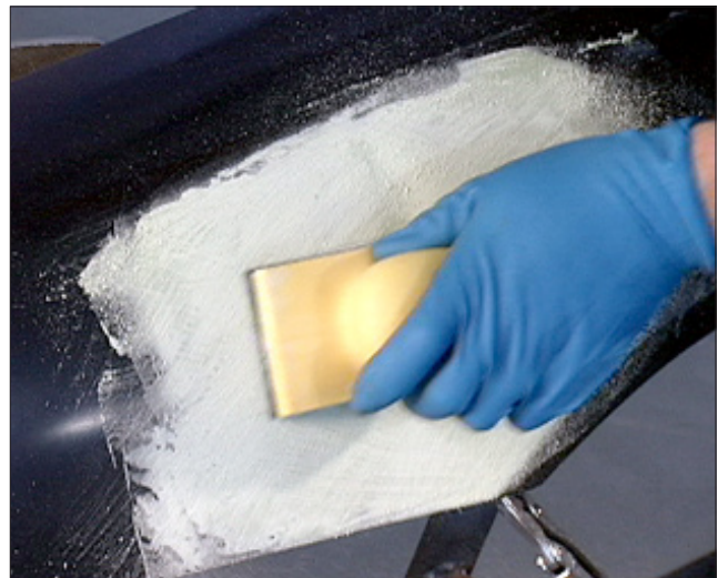
H-4 Use even pressure to sand the entire repair area.
