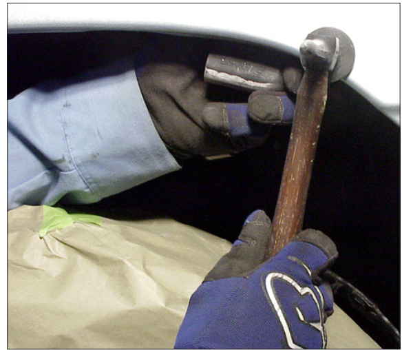
F-8 Changing the distance between the edge of the dolly and the face of the hammer makes the metal react differently.
