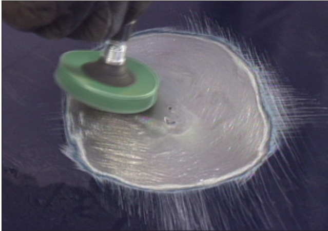
K-1 A plastic abrasive wheel may be used to remove the coatings without removing the metal in the repair area.
