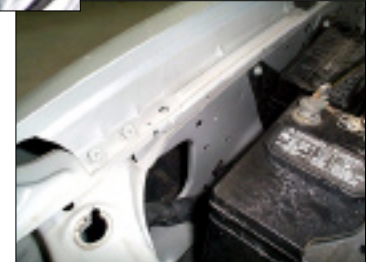
C-8 Access to the damage affect the methods that can be used to remove the damage.
