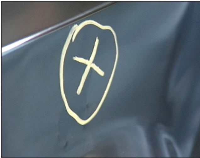
D-12 Notice the high spots in and around the circle.
