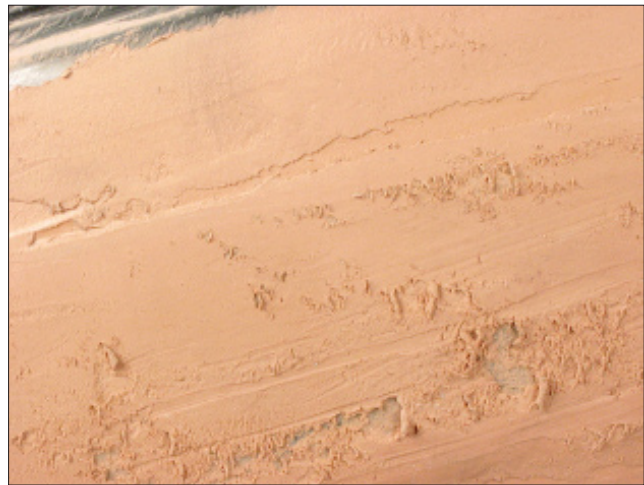
D-10 This body filler and hardener mixture began to cure before the technician was finished applying it to the repair area.
