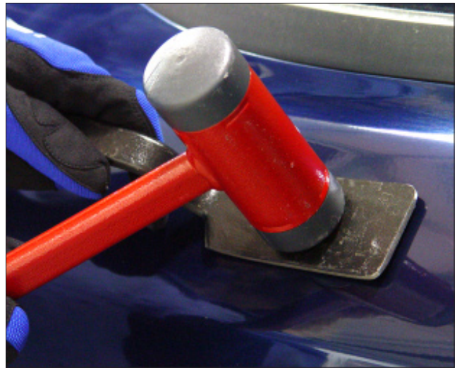
G-7 Both ball peen and dead blow hammers may be used to strike a spoon.
