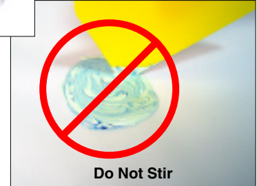
D-7 The spreader that is used to mix this body filler will not be used to apply it to the repair area.
