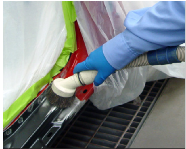
C-7 If large grinding particles are not removed before additional sanding, they could cause deep sand scratches.
