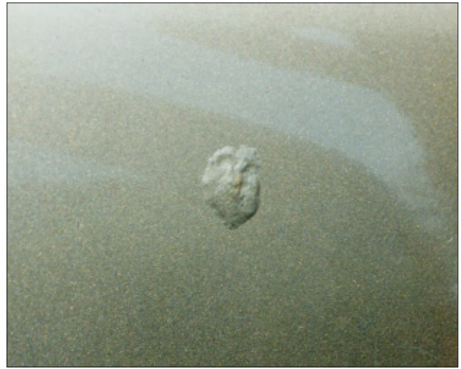
B-4 Corrosion will typically bubble under the paint before it breaks through and creates a hole.
